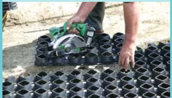
Panels can be cut to conform to shape using a handsaw or circular saw
