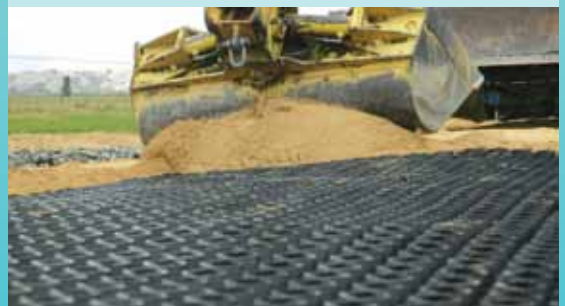
5+6. Fill SurePave with desired filling material to 20-30mm above top of panels and compact well
