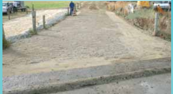
3. Compact well and spread a thin layer of "bedding material"
