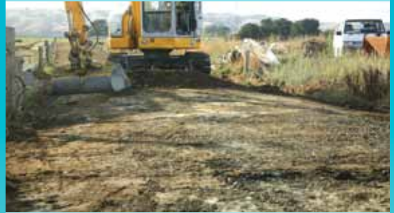
1+2 Create a clean, solid base with adequate falls
